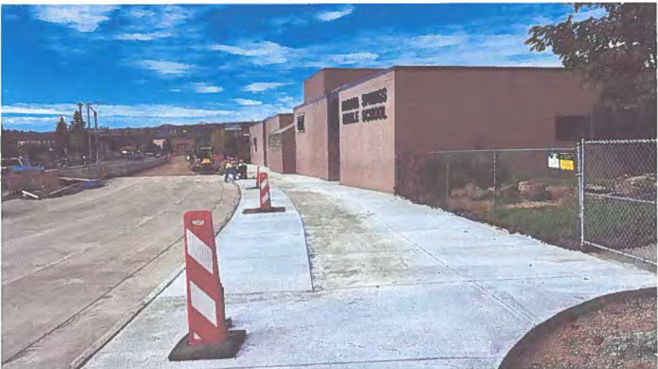
Pagosa Springs Middle School Sidewalk Project – In Progress
