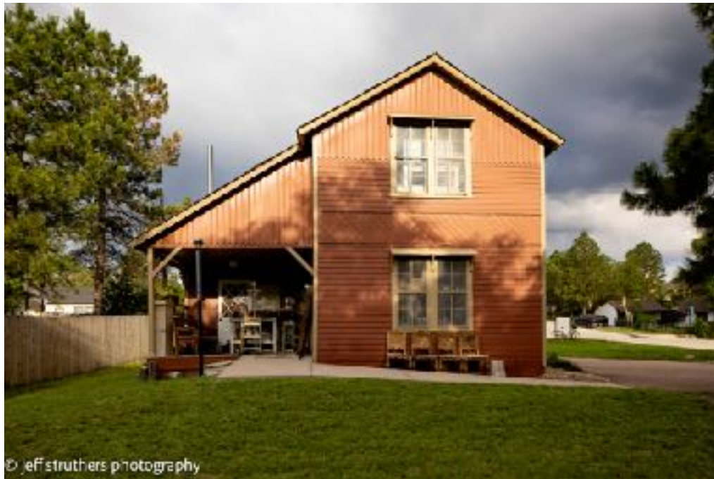
Section House at 338 Main Street, view from East.
